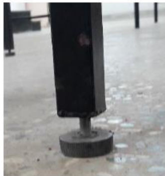
Height adjustment screw fixed to the bottom of the steel legs
